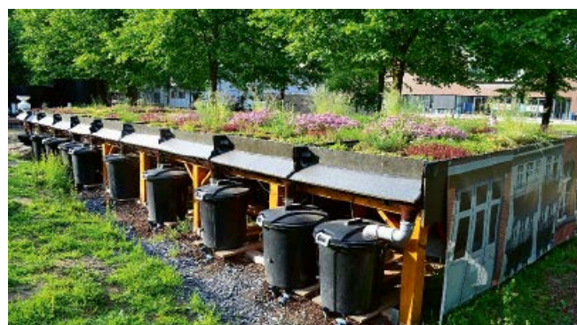
Fig. 1: Semi-technical test facility for extensive green roof structures
